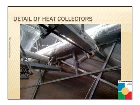
And hear we see a detail of the heat collector system, showing the mechanics needed to achieve tracking
