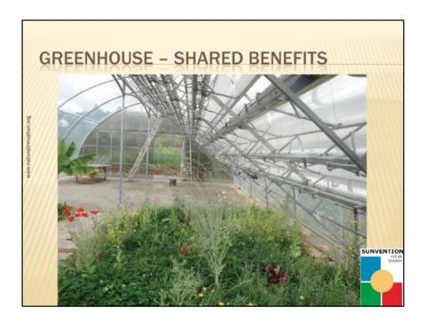
Looking inside you can see the horizontal lines are the heat collectors
